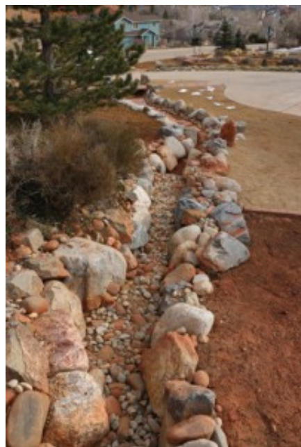
Dry creeks are very effective at channeling damaging water away from homes. (Photo by Wild By Design)
